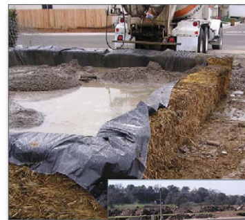
Figure 9. Hay bale and plastic washout pit
