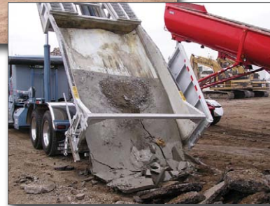
Figure 15. Delivering hardened Concrete to a recycler
