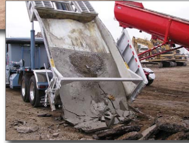
Figure 15. Delivering hardened Concrete to a recycler
