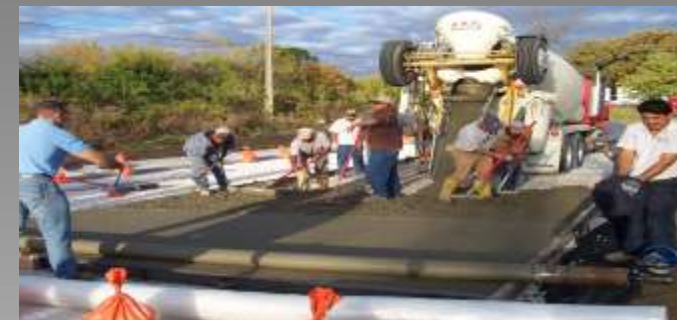
Specialized equipment is used to install pervious concrete.
