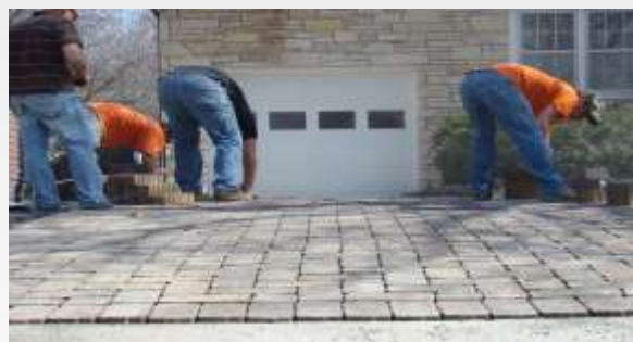
This homeowner in the Des Moines area had permeable pavers installed in the driveway.
