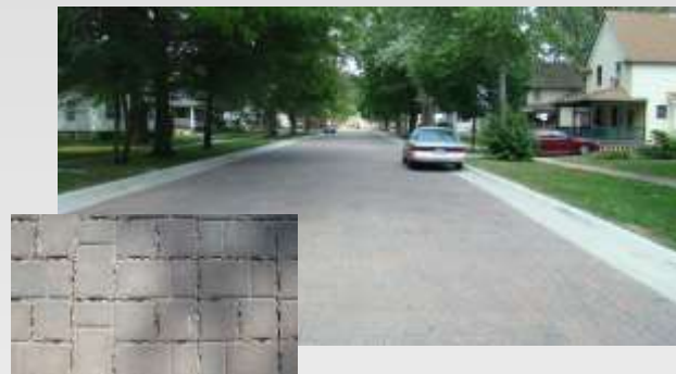
Charles City, Iowa has more than 25 blocks of permeable paver streets.
