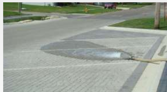
A demonstration of how water moves quickly into the spaces between pavers in a parking lot in West Union, Iowa.
