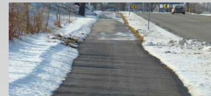
The sidewalk in the foreground is porous asphalt and drains faster than regular asphalt in the background.
