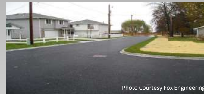
Porous asphalt street in Lake Manawa, Iowa.
